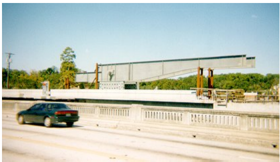
Figure 1 Trunnion-Hub-Girder (THG) assembly.
