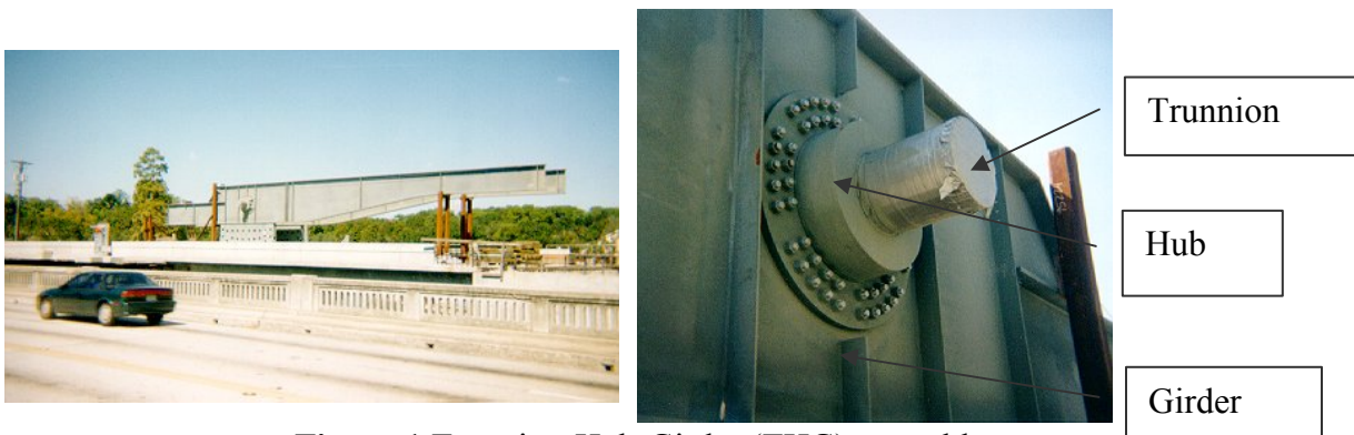
Figure 1 Trunnion-Hub-Girder (THG) assembly.
